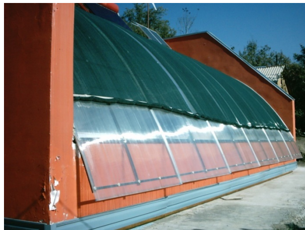
Photo 6 - Transparent fencing insulation of the experimental greenhouse from outside
